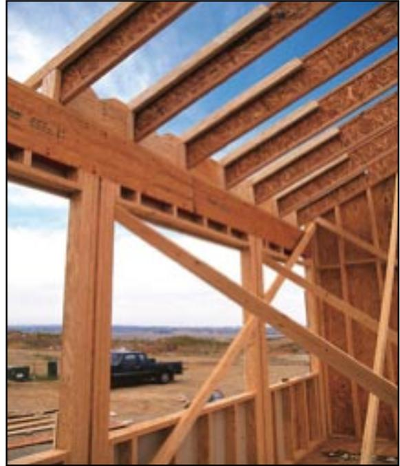
SCL is used here as a header above a window and as blocking between I-joists. Note the V-notches for roof ventilation.
