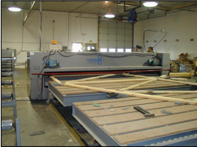
Figure 5 Truss Manufacturing Process
